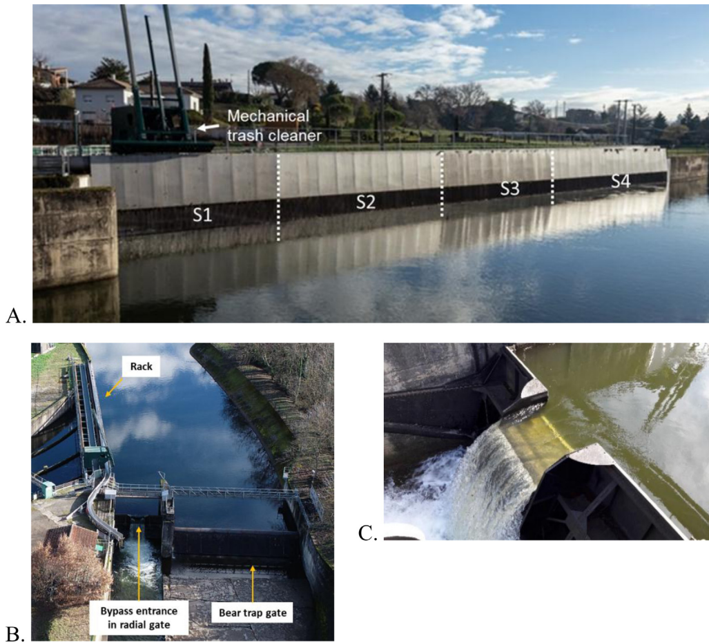
Fig. 2. A. Front view of the Pébernat 20 mm bar spacing rack, showing 4 sub-sections divided by downstream guiding walls, B. Downstream view of bypass entrance and bear-trap gate, C. Zoom on the bypass entrance created in the radial gate.
